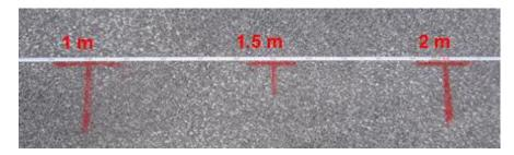
Figure 7-33: Marking grid line positions on the ground
